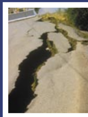
Many highways and roads could be made impassable by cracks and landslides following an earthquake.
