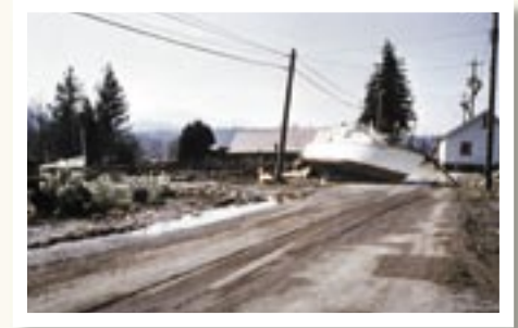
A tsunami struck B.C.'s west coast in 1964, causing extensive damage to Port Alberni and other communities in the area.
