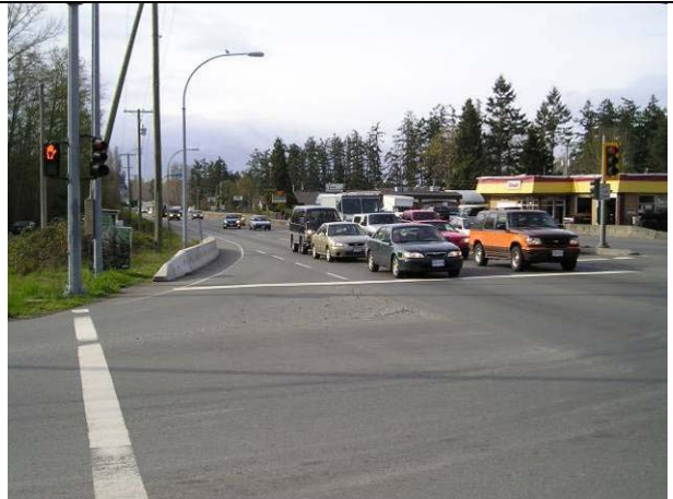
Hwy 17 Northbound approach: There is no designated right- turn lane from Hwy 17 to Sayward road; however, there is a paved triangle that may be used for right turns.
