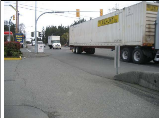
Hwy 17 Southbound, south of the intersection: Shell gas station accesses to Hwy 17 southbound are located close to the intersection.
