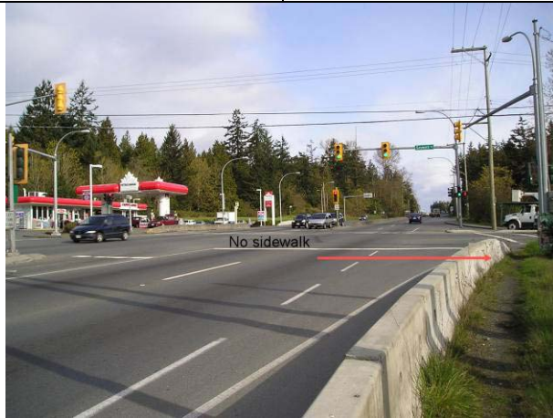
Hwy 17 northbound approach: there is no sidewalk adjacent to the northbound approach lanes. There is strong evidence of a pedestrian desire lane behind the barriers adjacent to the northbound lanes.
